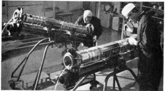
RESSED in surgeon's garb to assure complete cleanliness, technicians make final adjustments on new submarine telephone repeaters that "shoot" conversations across the bed of the Pacific Ocean. Built by a British affiliate of International Telephone and Telegraph Corp., these gold plated "guns" am-
