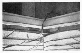
FIG. 6: Route the twinlead away from rain gutters and metallic masses. Use screw and nail standoffs.
