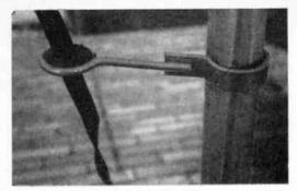
FIG. 7: Don't tape the twinlead to the mast. It's a sure way to lose some signal. Standoff shown snaps on.
