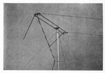
FIG. 5: Note that in the above installation, the mast is supported with guy wires and the twinlead is twisted to prevent whipping. Whipping often causes trouble.
